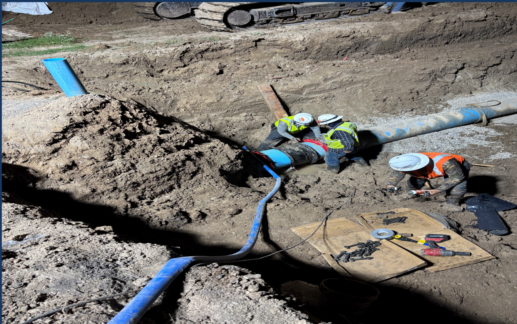
S. CAGE 18" WATER LINE RELOCATION STA. 1087+93
